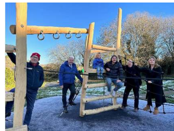
In December we concluded the refit of Collapark in Totnes – using S106, District and Town Council Contributions
